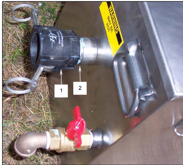
Figure 1. Replacing the Grease Separator Inlet Coupler.
