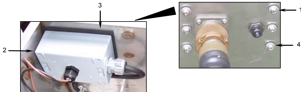
Figure 5. Installing the Grease Separator Weatherproof Box.
