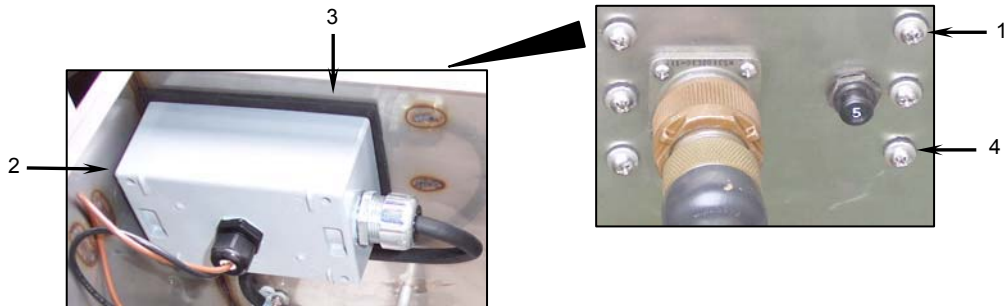
Figure 6. Installing the Grease Separator Weatherproof Box.
